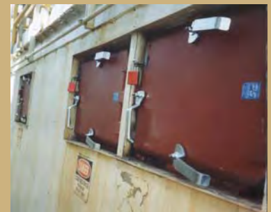
Standard Access Hatches With Hasp Locking Device.
